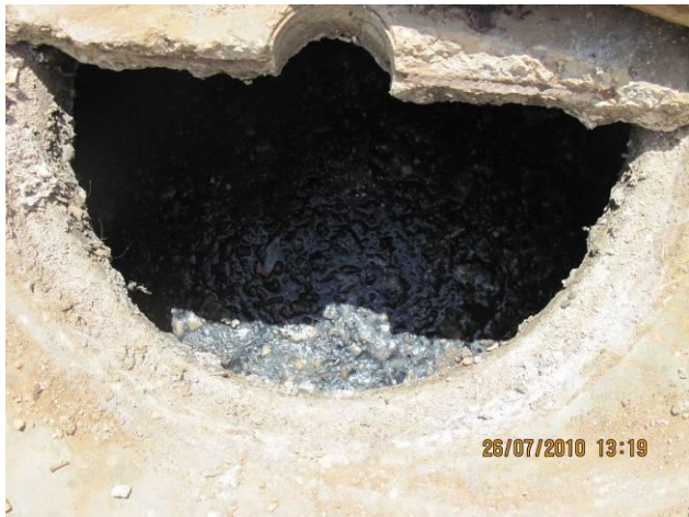
Photo B.6 Collective onsite Upflow Gravel Filter wastewater treatment plant in Al Mazr'a Al gharbiya Village in Ramallah Governorate. Right photo shows broken cover of septic tank.
