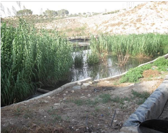
Photo B.2 Community onsite wastewater treatment plant consists of Up-flow Anaerobic Sludge Blanket (UASB) - Horizontal Flow Constructed Wetlands located in Nuba Village in Hebron Governorate. The right photo shows a penetration on the borders of Constructed Wetlands which leads to infiltrates the sewage into the surrounding layers and does not reach the effluent storage tank
