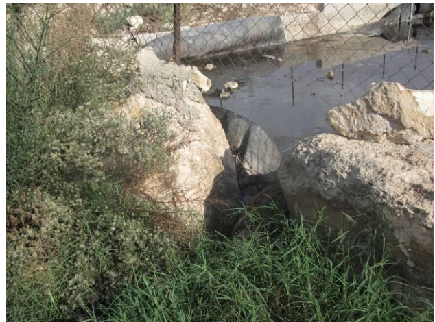
Photo B.2 Community onsite wastewater treatment plant consists of Up-flow Anaerobic Sludge Blanket (UASB) - Horizontal Flow Constructed Wetlands located in Nuba Village in Hebron Governorate. The right photo shows a penetration on the borders of Constructed Wetlands which leads to infiltrates the sewage into the surrounding layers and does not reach the effluent storage tank
