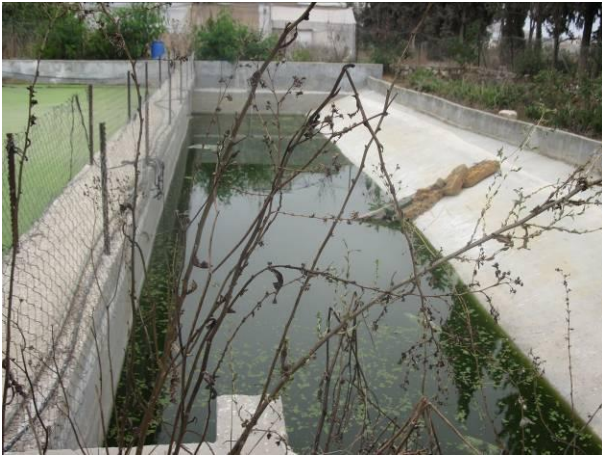
Photo B.5 Collective onsite wastewater treatment plant consists of Duckweed-based pond system located at Al Aroub agriculture school in Hebron Governorate
