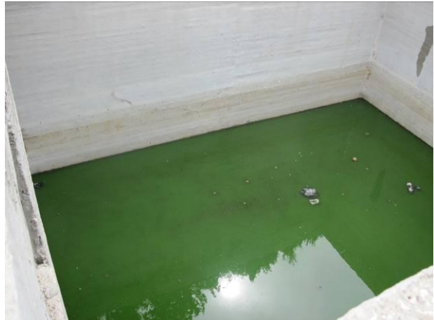
Photo B.5 Collective onsite wastewater treatment plant consists of Duckweed-based pond system located at Al Aroub agriculture school in Hebron Governorate
